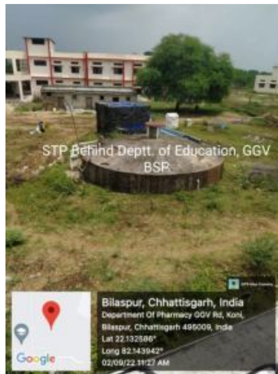
STP behind Department of Education
